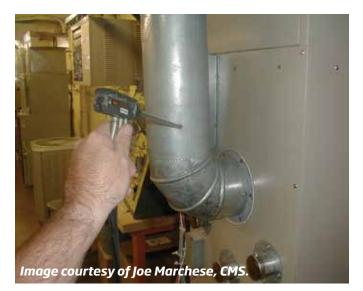
Combustion analyzers take a continuous sample of flue gases to quickly report changing burner conditions.
